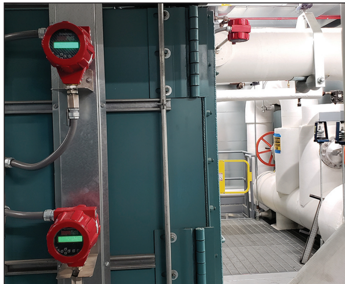
Figure 6. Insertion multivariable vortex mass flowmeters measure steam—one process connection for mass flowrate, temperature, pressure, volumetric flowrate, and fluid density simultaneously.
